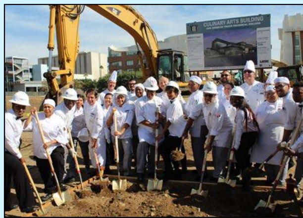
LATTC Culinary Arts Building Groundbreaking.
