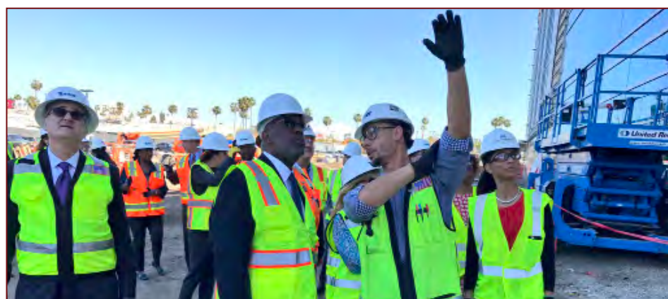
Noah Boro, Superintendent at Turner Construction Company, describes the construction of the new Kaiser Permanente Baldwin Hills-Crenshaw medical facility to CEO of Kaiser Permanente, Bernard Tyson.
